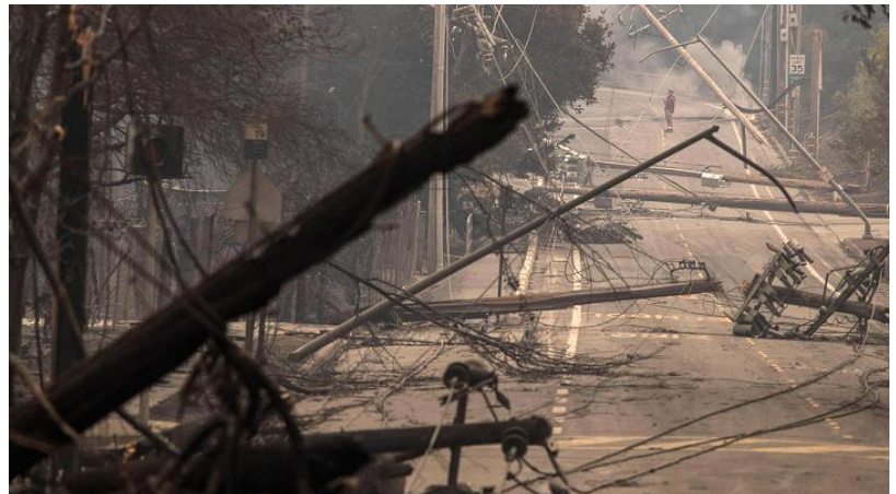
Image 1: Downed power poles and lines in 2017 Fire Siege
