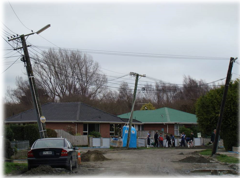
Picture: Leaning Poles due to February 2011 Christchurch Earthquake. Source: http://thunderboltz.blogspot.com
