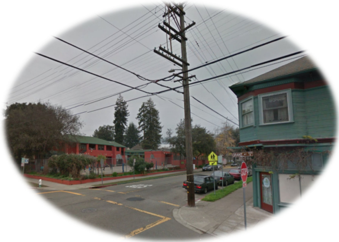
Picture: Utility Wires at Grant and Bancroft. Source: Berkeleyside.com
